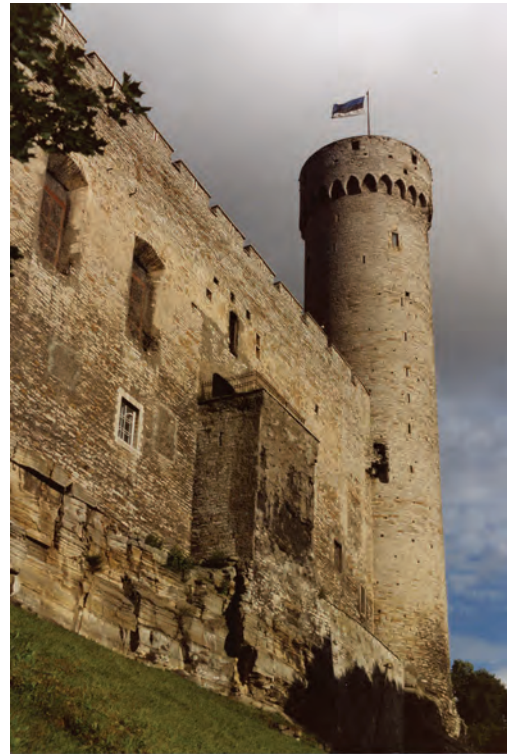
Fig. 23. Centre of the Old Town of Tallinn, the Toompea Hill, is a klint island. The Building Limestone (Vão Formation, Darriwilian) from the klint and adjacent areas has been extensively used in buildings of the Old Town, which was inscribed in the World Heritage List in 1997. Photo by J. Nölvak.
