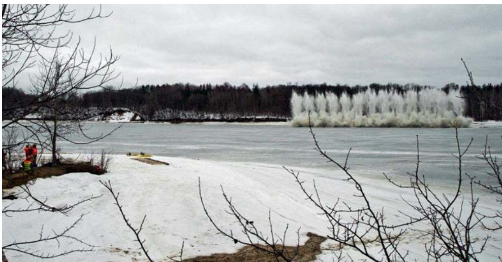
Figure 84. Ice blasting on Daugava River near Pļaviņas HPP
