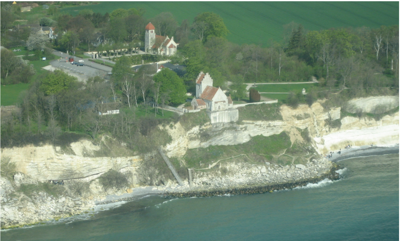
Figure 8. The landslide at Højerup old church. The top of the landslide body is c.15 m a.s.l. and the toe of the slide is protected against erosion with blocks and boulders. The new church in Højerup was built in 1913 due to the local fear for destruction of the old church by a landslide.
