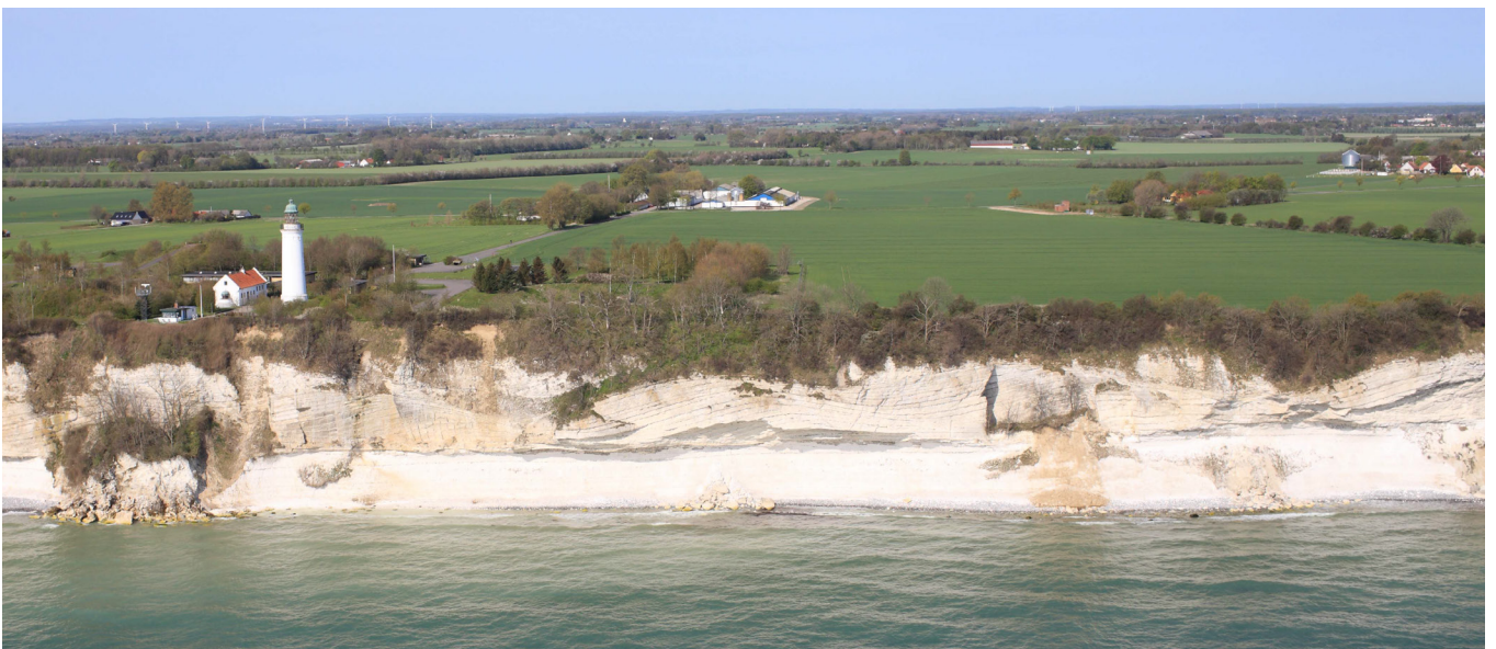
Figure 6. Photo of the cliff-fall and the large overhang at Stevns Fyr. The lighthouse is located at the highest point along Stevns Klint, 41.5 m a.s.l. Below and north of the lighthouse the rectangular shaped small limestone quarries can be seen. Note that under the substantial overhang a small pile of blocks indicate a rock-bedding exfoliation of the roof below the overhang. This type of erosion contributes to the decrease in the thickness of the overhang, which decreases its strength and thus increases its tendency of a cliff-fall (or cliff-slide).
