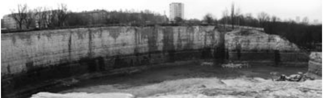
Excavation of the new Museum of Art in Tallinn provided an excellent outcrop for Ordovician research. Photo by G. Baranov.
