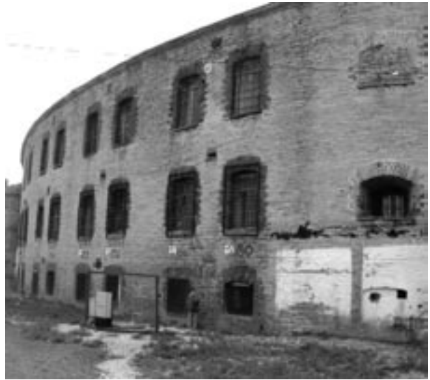
The former city prison is a typical limestone building in Tallinn. It is made of Ordovician limestone of the Vão Formation. Photo by G. Baranov.
