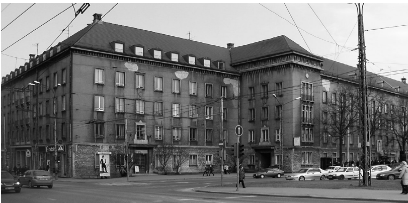
Main entrance of the building at Estonia Ave 7, hosting our institute since 1952. In summer 2006 the Institute will relocate to the campus of the Tallinn University of Technology in Mustamäe.
