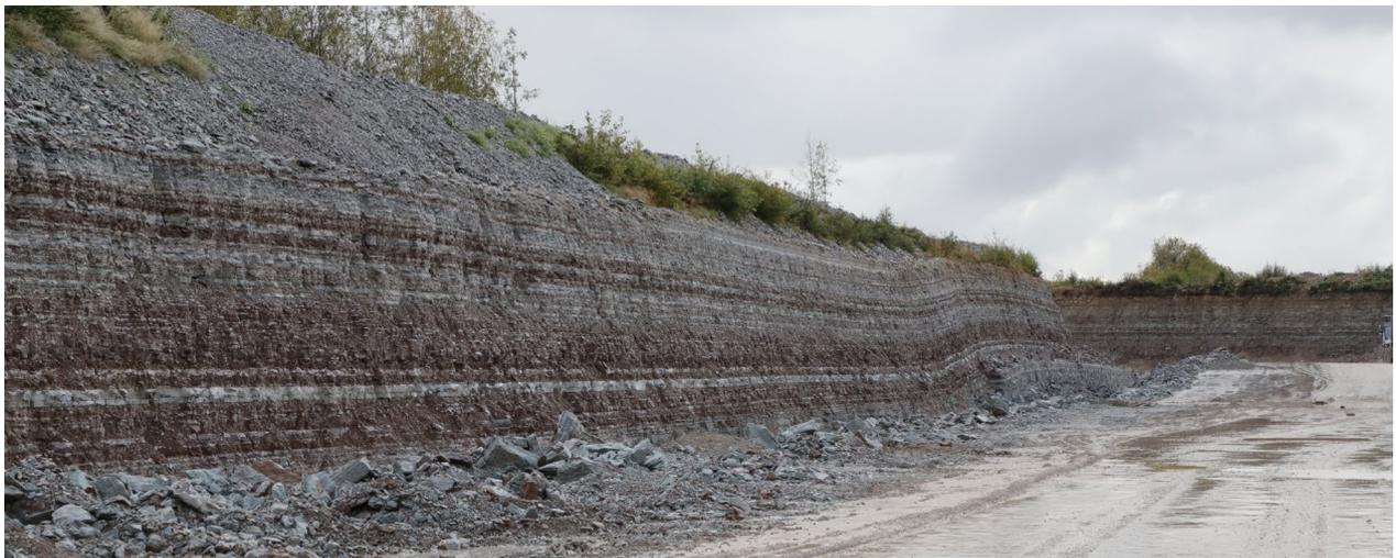
**Fig. 4.2.** Oil shale succession in the Põhja-Kiviõli II open-pit mine. Photo: Gennadi Baranov, 2019.
